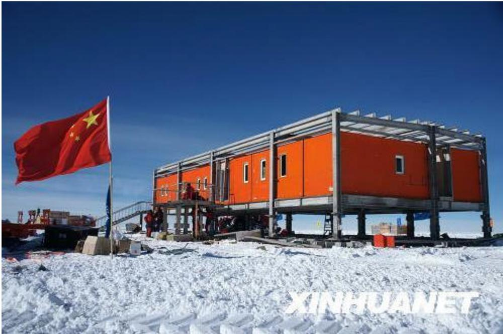
China's 25<sup>th</sup> Antarctic expedition team said on January 15, 2009 that it has completed the framing part of building a new station in the Antarctica, with 11 cabins in the place. Kunlun station will be built with pre-fabricated components and on-site installation. The steel frames have been erected on the selected site, and walled with insulation boards. To keep the temperature right for residence, even the container like cabins are walled with insulation boards.
