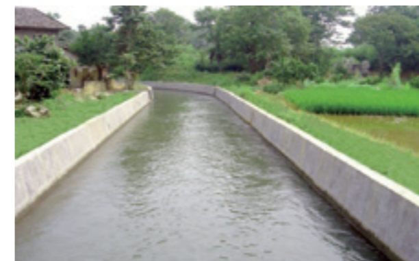
A renovated canal in the irrigation area at Liuchen, Guangxi Province
